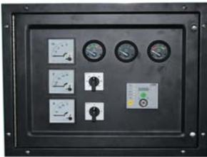
The Model 702 is a Manual Engine Control Module designed to control the engine via a key switch and pushbuttons on the front panel. The module is used to start and stop the engine and indicate fault conditions, automatically shutting down the engine and indicating the engine failure by LED, giving true, first up fault annunciation.
