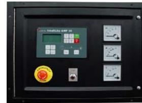
The AMF25 is an Automatic Mains Failure module with generator monitoring, protection and start facilities. The controller has a large LCD screen, display the generator's each parameter, running and alarm information. The off/replacement button, mode switch button, start/stop button and the LED indicator light, makes the user easy to operate and maintain the generator.
